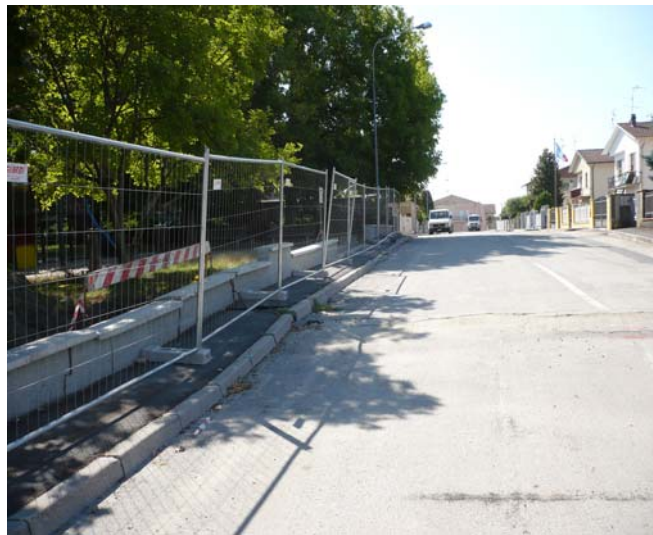
Fig. 4. The difference in level that appeared in the village of San Carlo after the mainshock of 20 May 2012.
